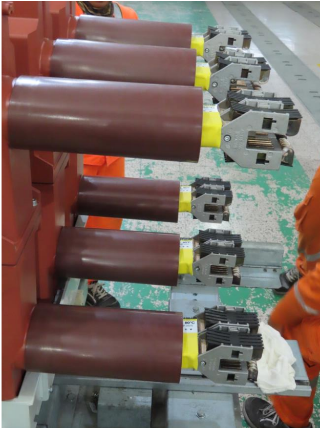
Withdrawable contacts loosen with number of operations
