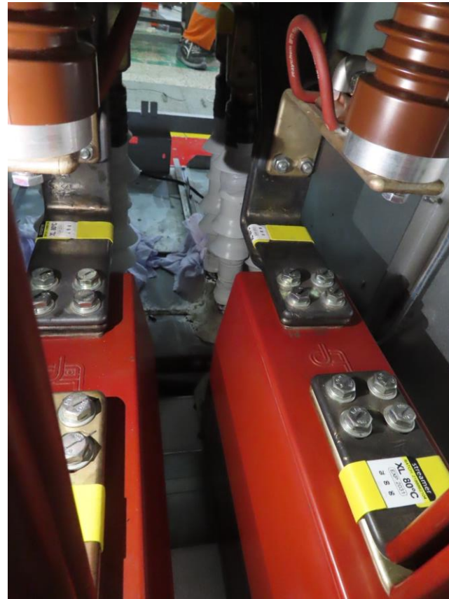
Withdrawable contacts loosen with number of operations
